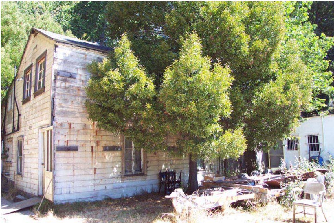
South elevation, 1102 10 th Street
