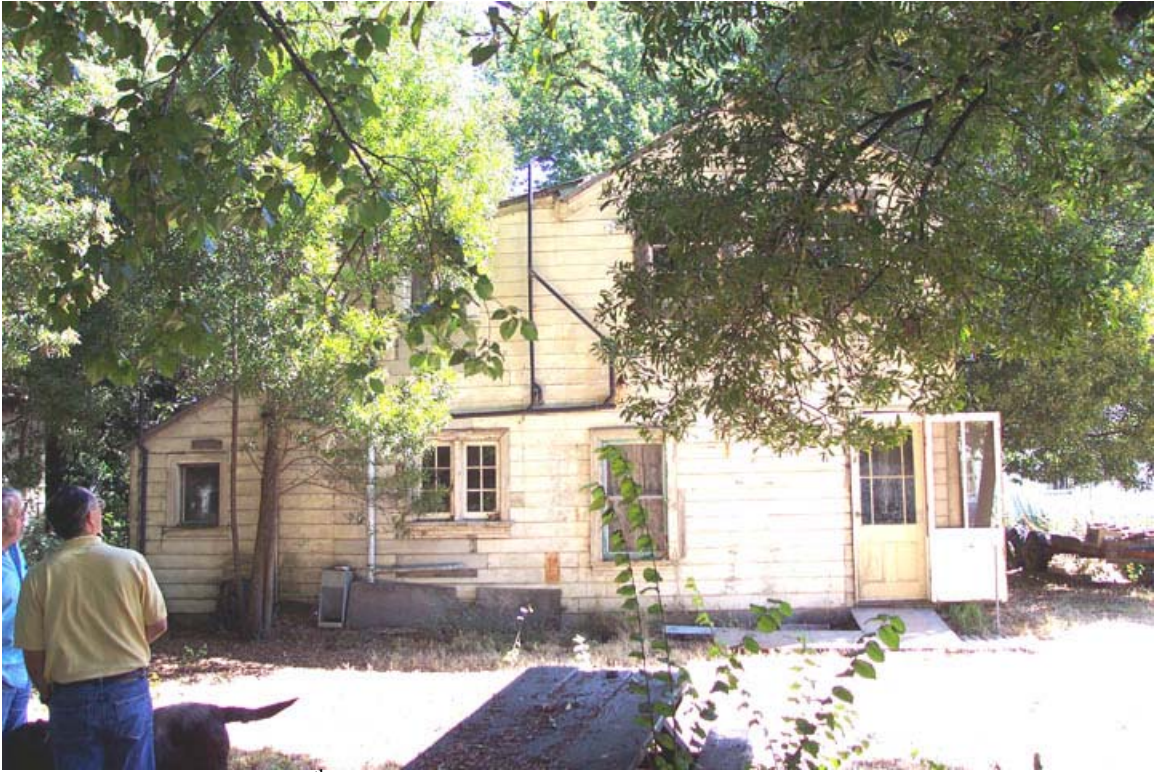
West elevation, 1102 10 th Street
